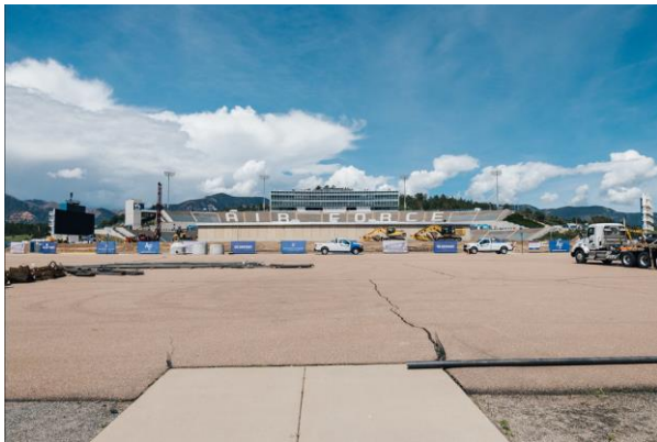
East side upper stands/entrance removed
